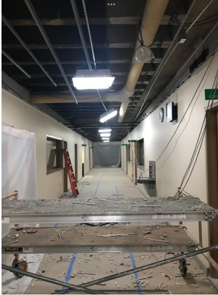
New lighting and HVAC work was installed throughout the Administration wing of the Courthouse.
