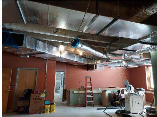
New lighting and HVAC work was installed throughout the Administration wing of the Courthouse.
