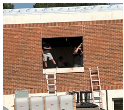
The older windows were replaced with windows that would be a lot easier for staff and residents to open.
