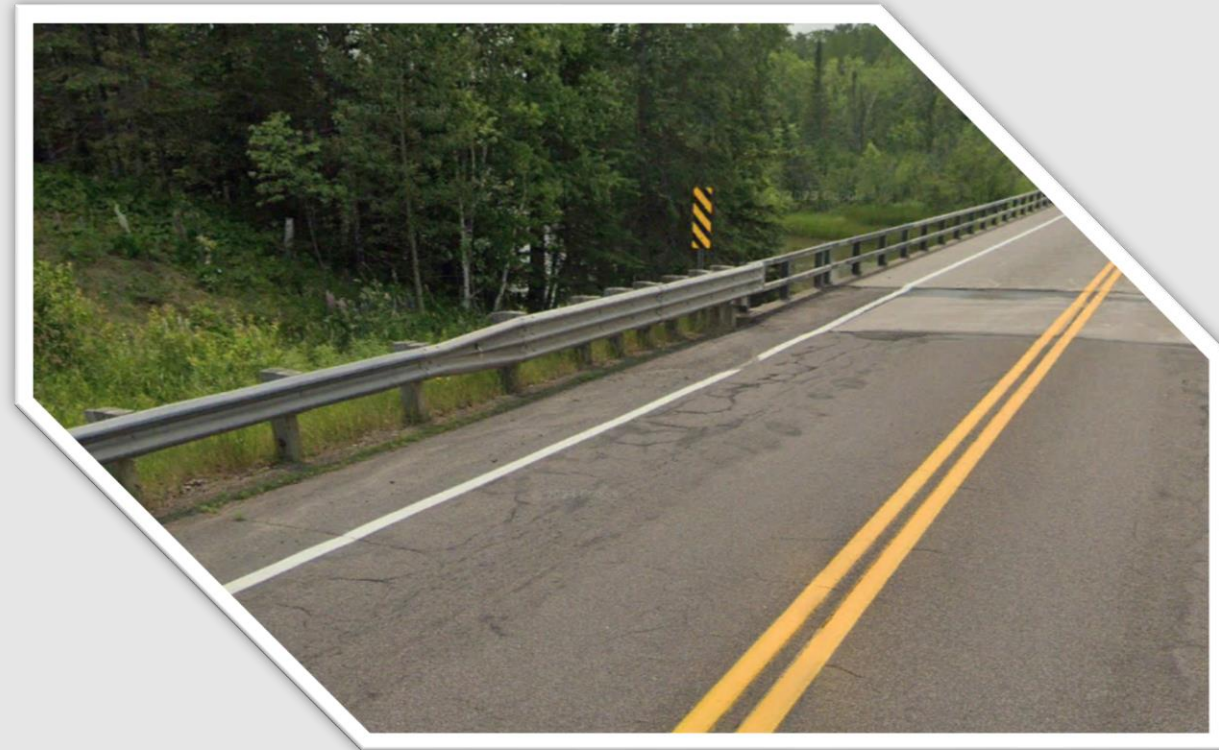
Iron River Bridge approach
